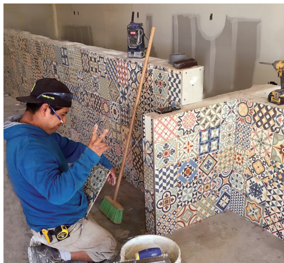
A Handian Construction professional carefully installs decorative Mexican tile at Lola's Mexican Cuisine in Long Beach, Calif.
